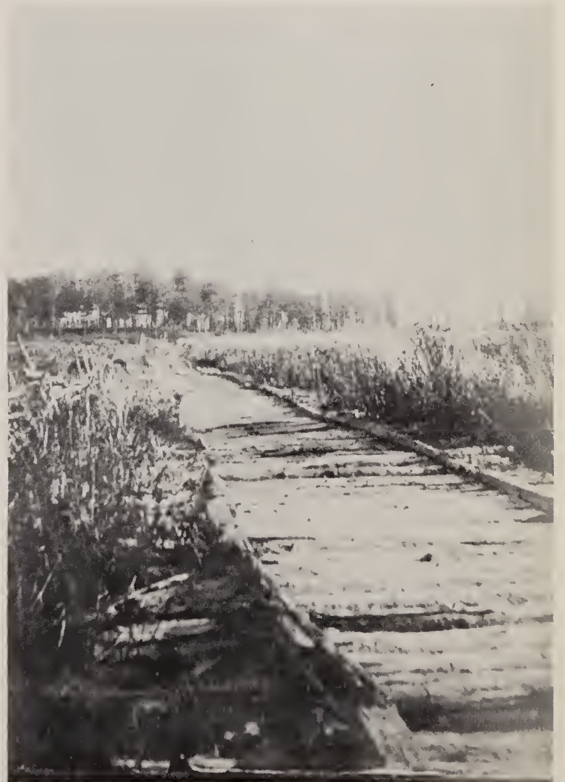
PLANK CAUSEWAY AND FLOATING BRIDGE TO STROEBE'S ISLAND, 1900
