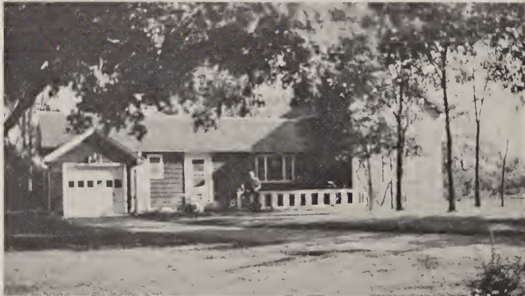
THE HARRY STROEBE, SR., HOME, 1945 on the north half of the island.
